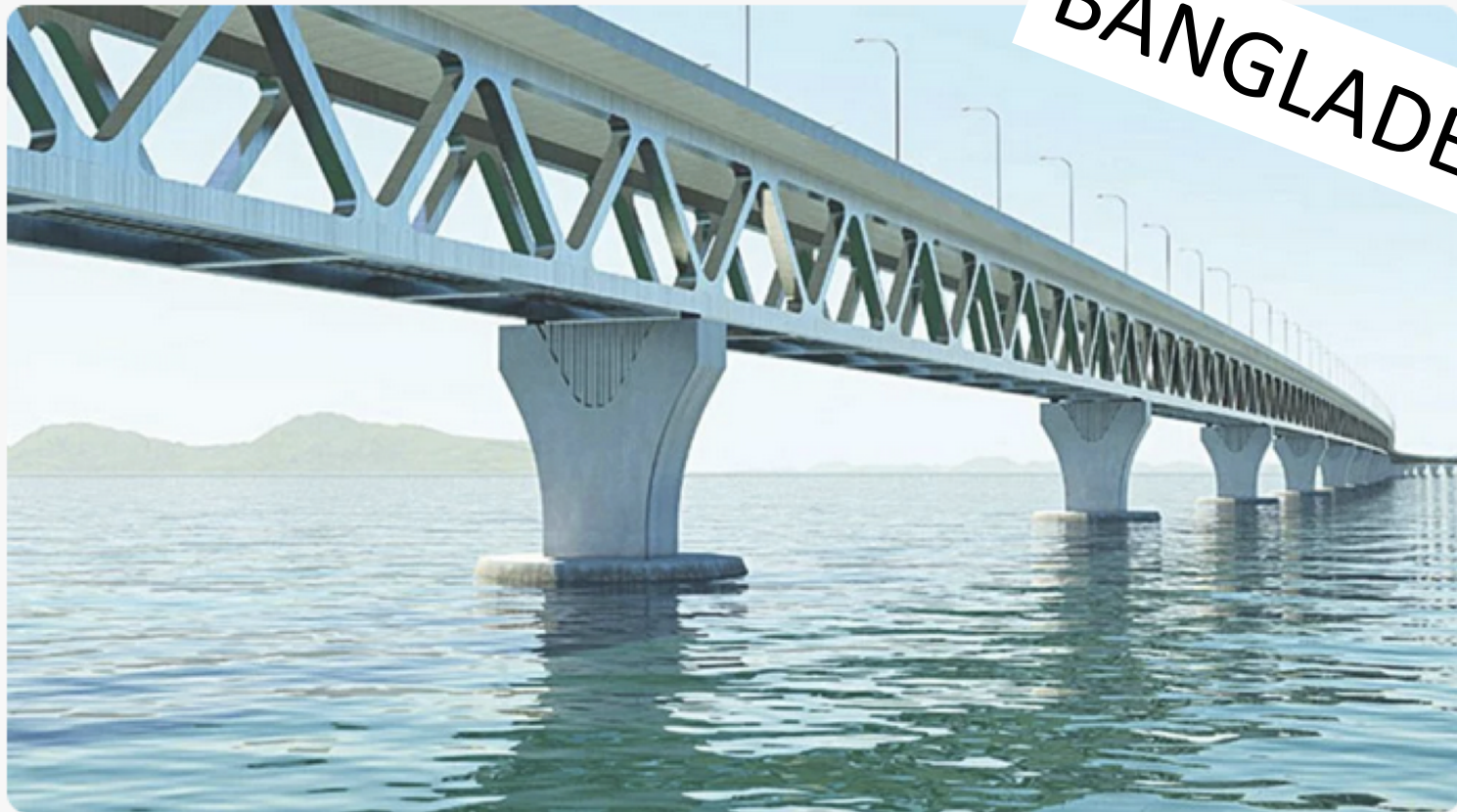
Photo: Padma Bridge (Under Construction), Padma River – Bangladesh.
