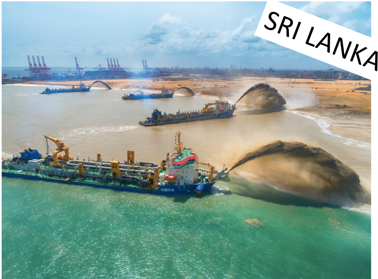
The land reclamation project in Colombo, Sri Lanka, jointly undertaken by China Communications Construction Co. Ltd. and the Sri Lankan Government under the Belt and Road Initiative. Completed on January 16, it reclaimed 269 hectares of land in less than three years (XINHUA)
