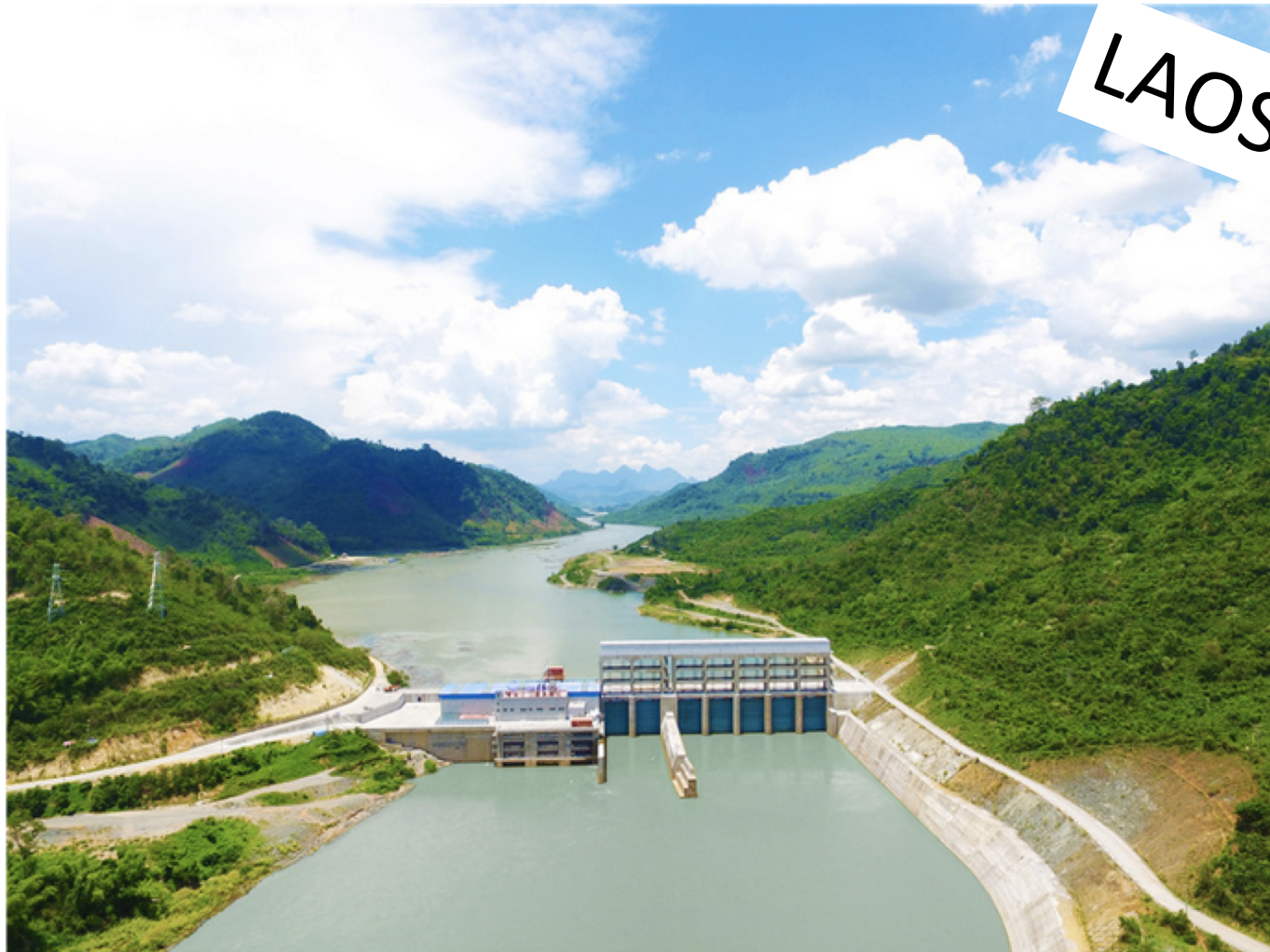
The level-2 station of the Nam Ou project has been in operation since 2016. The project, with an installed capacity of 1,272 megawatts, is invested in and constructed by Power Construction Corp of China at a cost of $2.73 billion. Provided to CHINA DAILY
