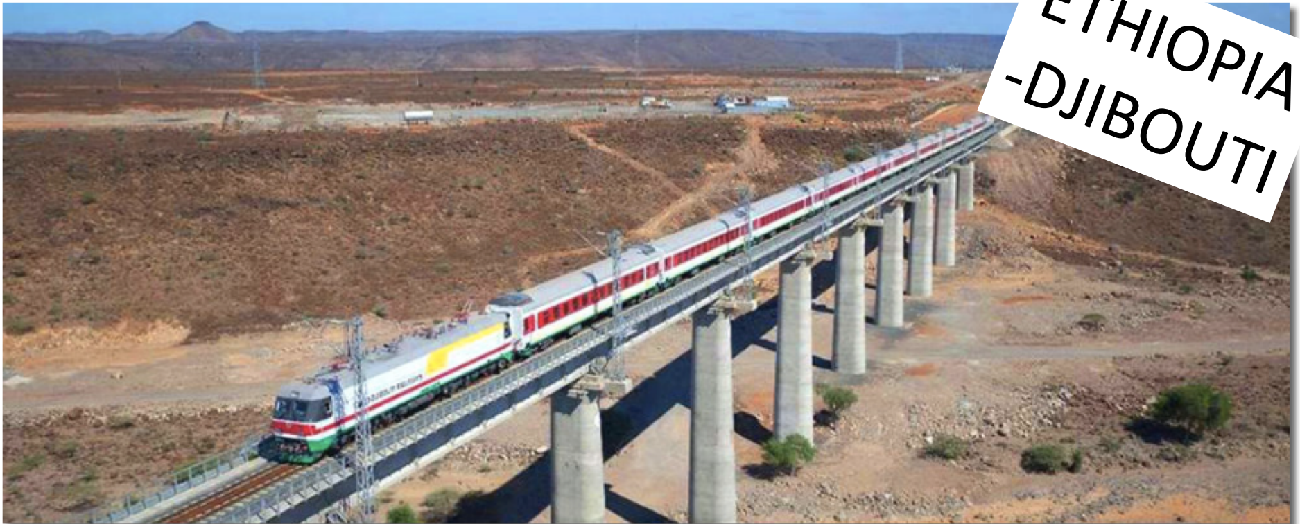
The Chinese-built Addis Ababa–Djibouti Railway. (Photo: Skilla1st )
